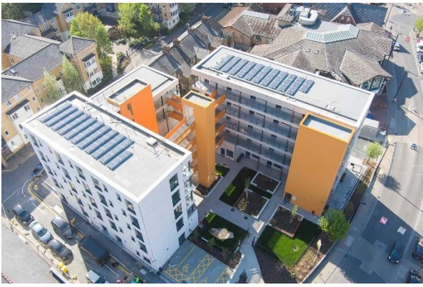
Bridge Court, Desborough Road – Exterior (Premier Modular)
